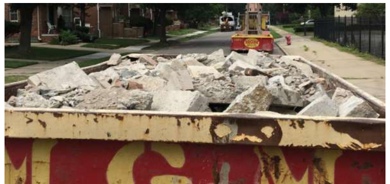
Four dumpsters of concrete removed to create gardens
