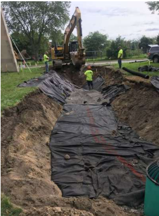
Construction of the East bioswale
