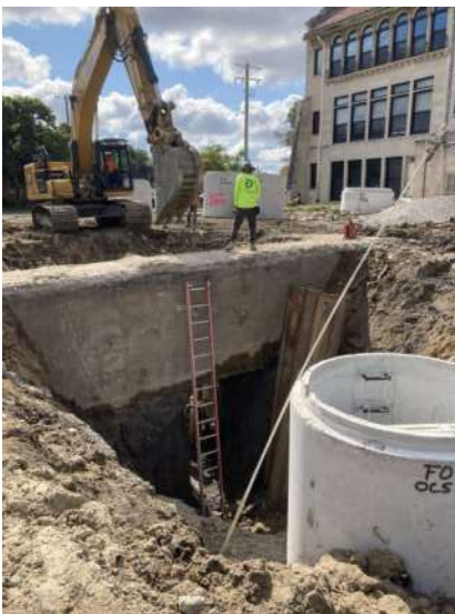
Underground storage being prepared to detain water runoff
