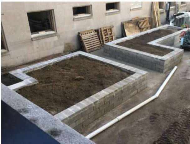
Above ground gardens constructed
