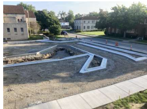
Curbing added to direct waterflow
