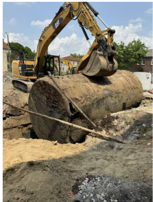
An excavator lifts the tank out of the ground
