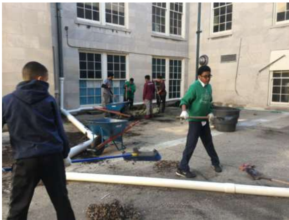
Cleaning the courtyard before construction
