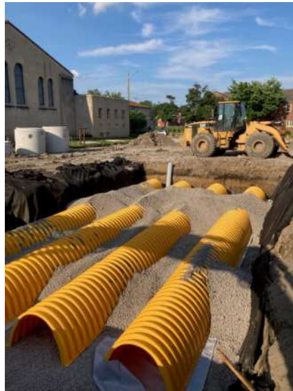
Underground storage being prepared to detain water runoff
