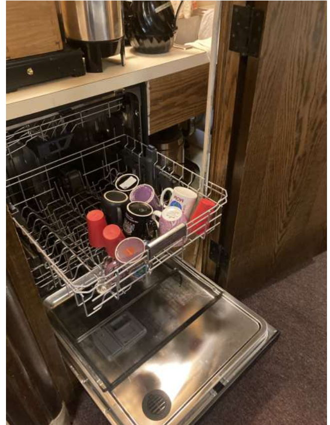
Newly installed dishwasher
