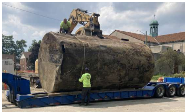
The tank was loaded onto a semi truck and hauled away
