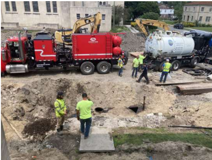
The tank was located and the oil needed to be heated before it could be siphoned out of the tank into tanker trucks
