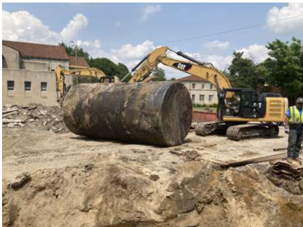
Moving the oil tank was an onerous project
