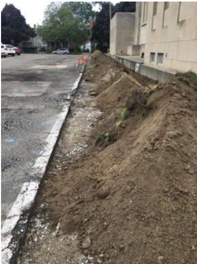
Dirt placed over concrete
