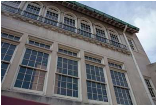
Original single paned windows
